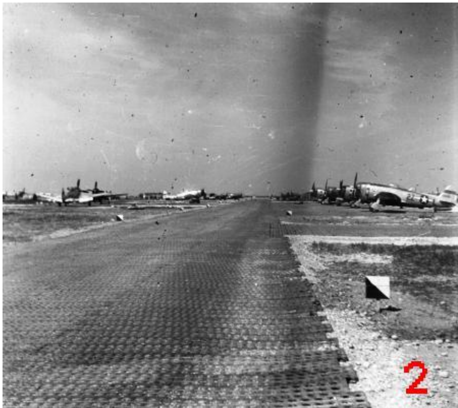
Image 1: The building is Bure Homage House. This was used as an Officers Mess by the 405FG. After the war used for a time by the Royal Signals and demolished in 1957. Image 2: A view looking along the Pierced Steel Planking taxiway.
