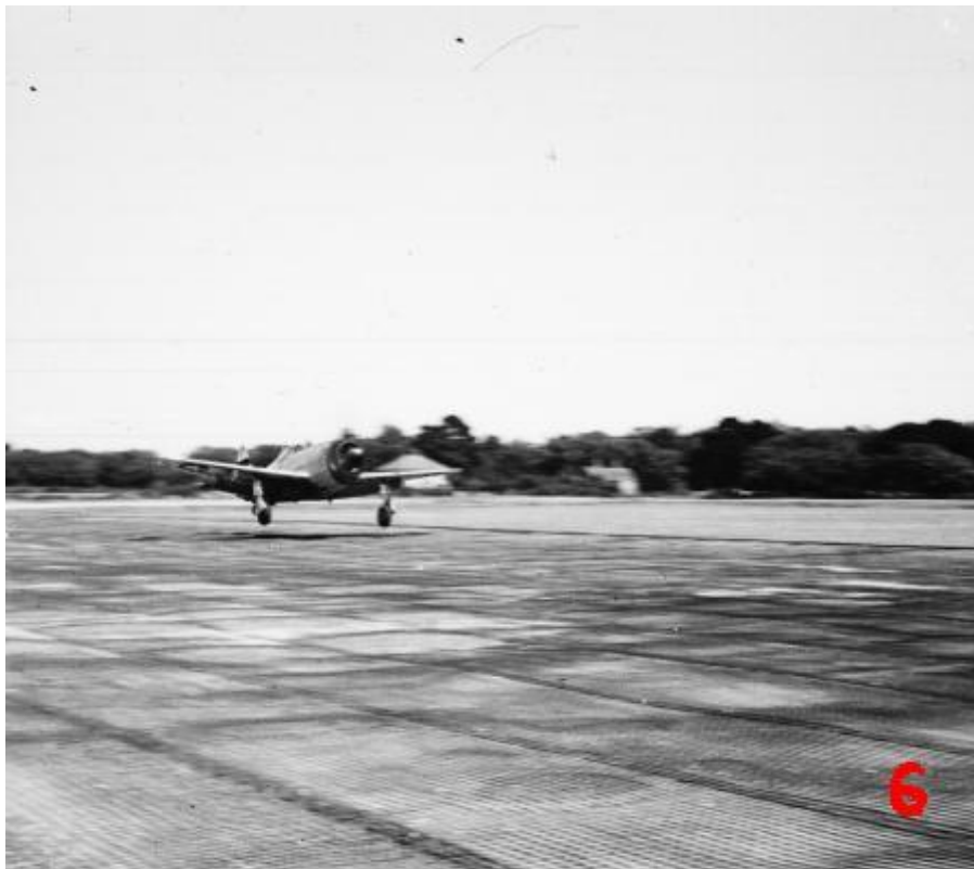
Image 5 shows the tented accommodation used by the 405th. Image 6 - A P47D landing on the Steel Matting Runway.
