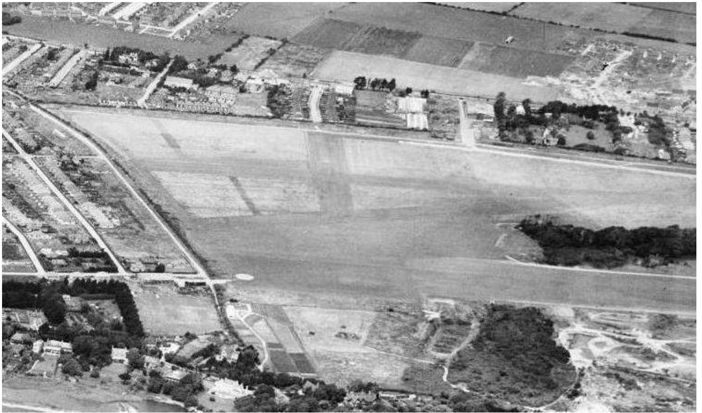
The picture above shows the western end of the aerodrome in 1950.
