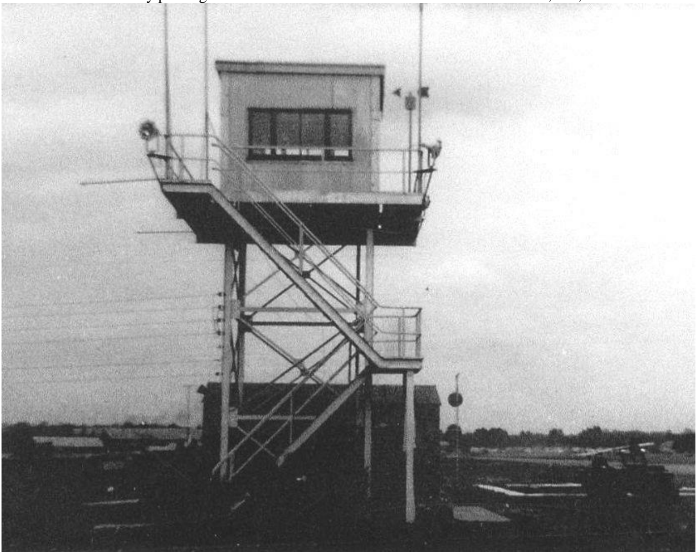
Christchurch Control tower.
