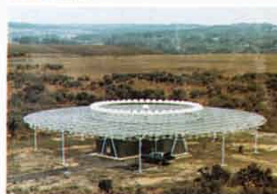
A DVOR radio beacon
