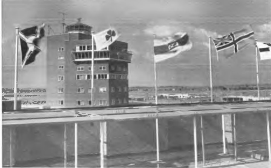
The Control Tower
