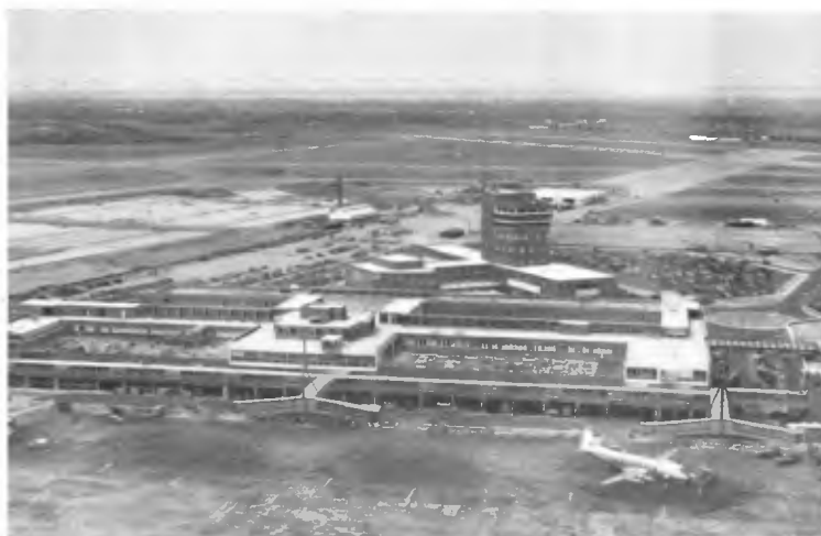
General View of the Control Tower and Passenger Building
