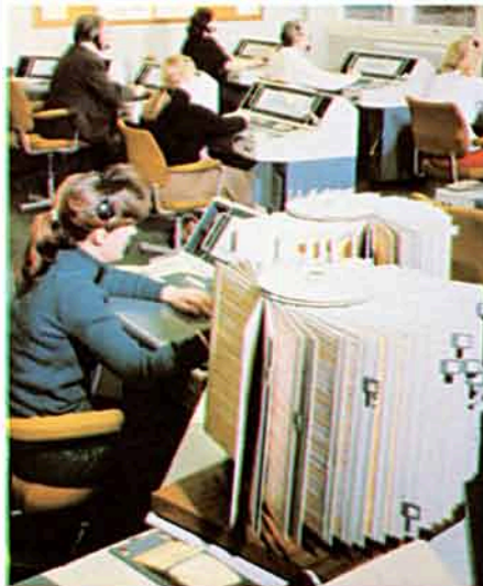
Above The airport telephone room
