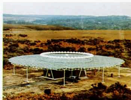
A Doppler VHF omni-directional radio beacon used by aircraft to navigate to and from Heathrow
