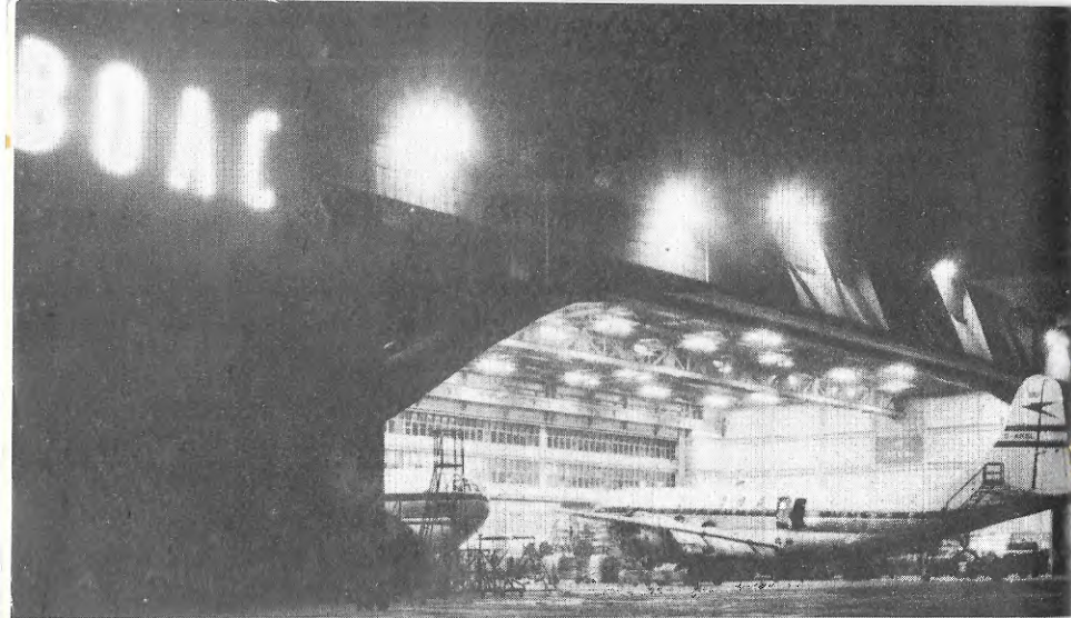
Night Maintenance BOAC Headquarters.
