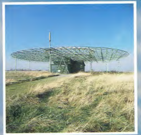
A Doppler VHF Omni-Directional radio beacon which transmits navigational information to pilots
